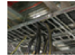
Swifts cable ladder: main distribution infrastructure
