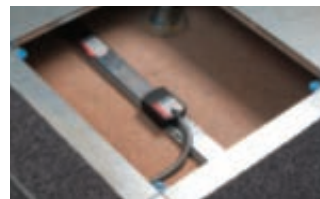
Electrak busbars
